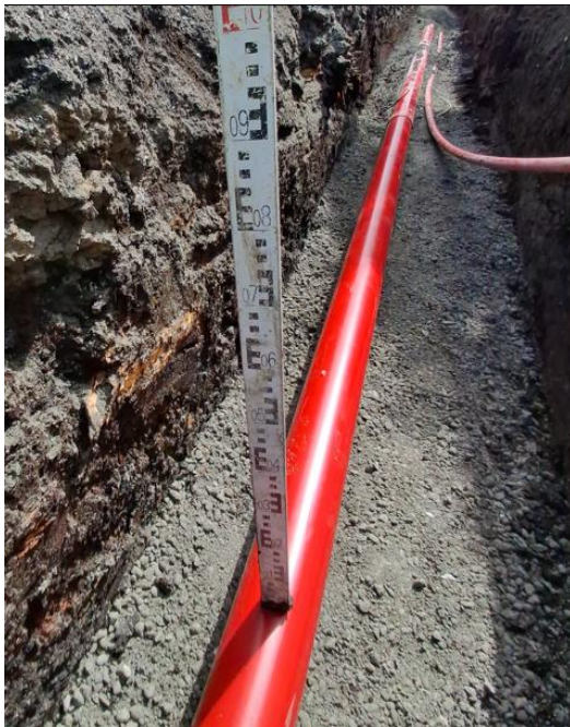
Plate 2-1 Typical Single Cable Trench View
